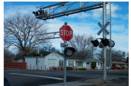
*Figure 6 Crossing with Flashing Light and Crossbucks*
