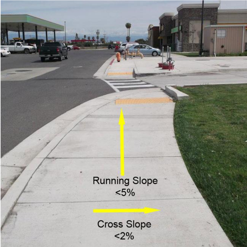
Figure 1: Illustrating cross and running slope measurements
