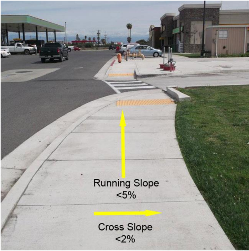
Figure 1: Illustrating cross and running slope measurements
